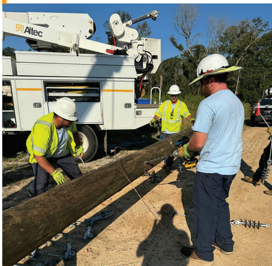
Linemen replacing broken poles from the storm damage.
